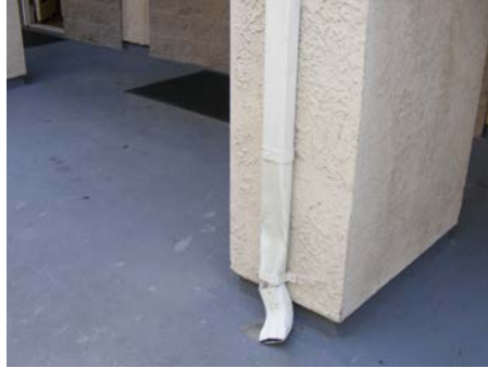
Crushed Downspout
