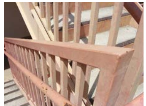
Exterior Guard Rail Condition, Typical
