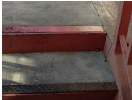
Exterior Stair Condition, Typical
